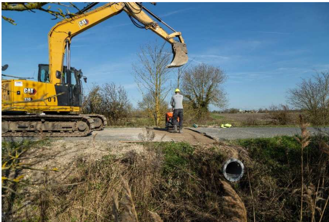
Figure 15: installation de la buse
