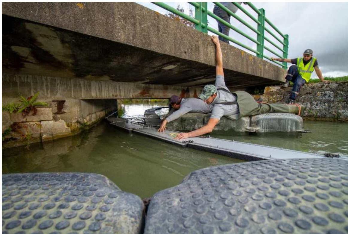
Figure 14: installation des pontons
