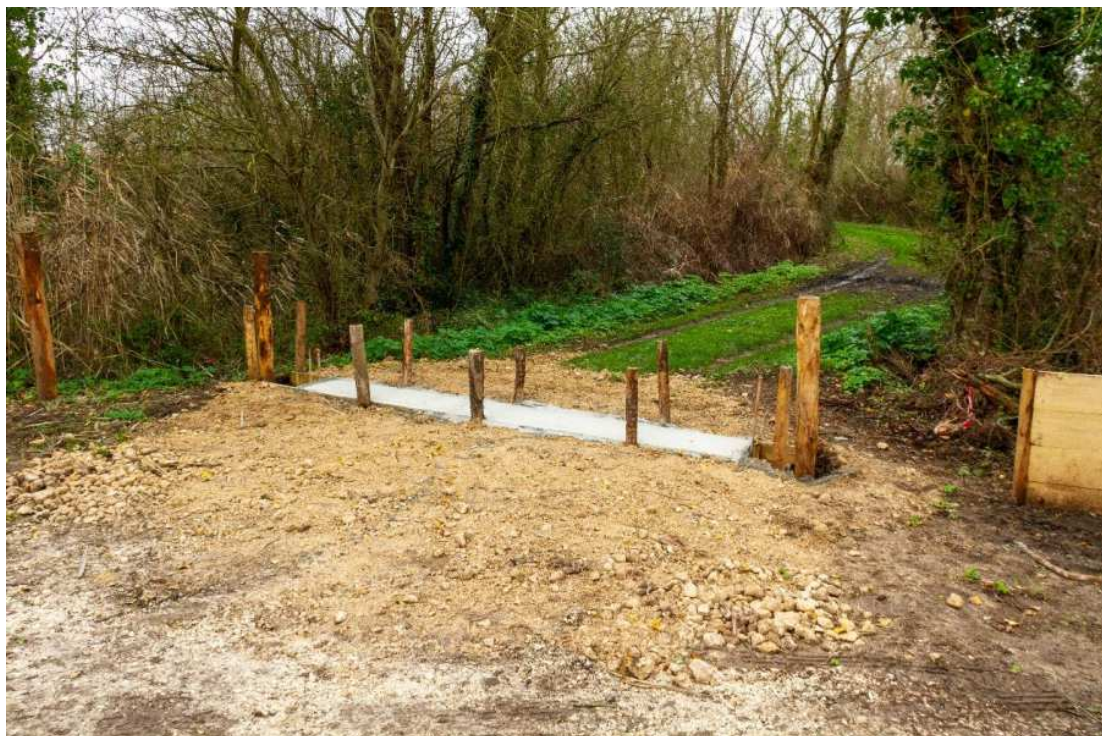
Figure 25: coulage de la longrine
