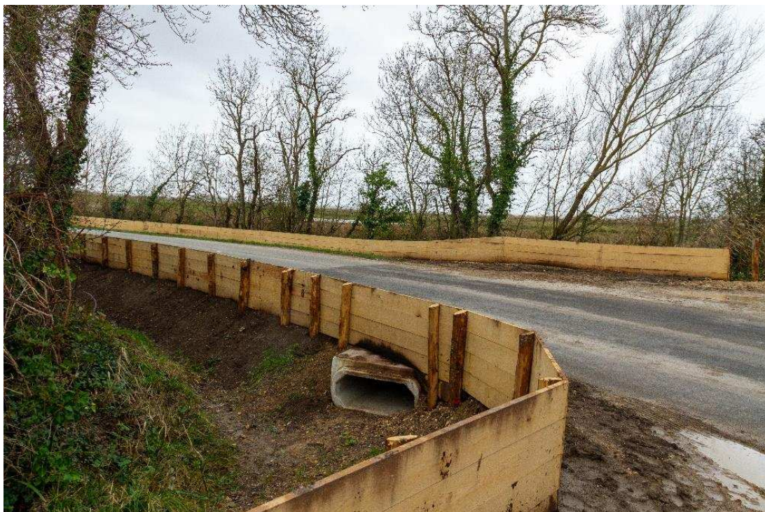
Figure 22: finitions et raccordement aux dalots
