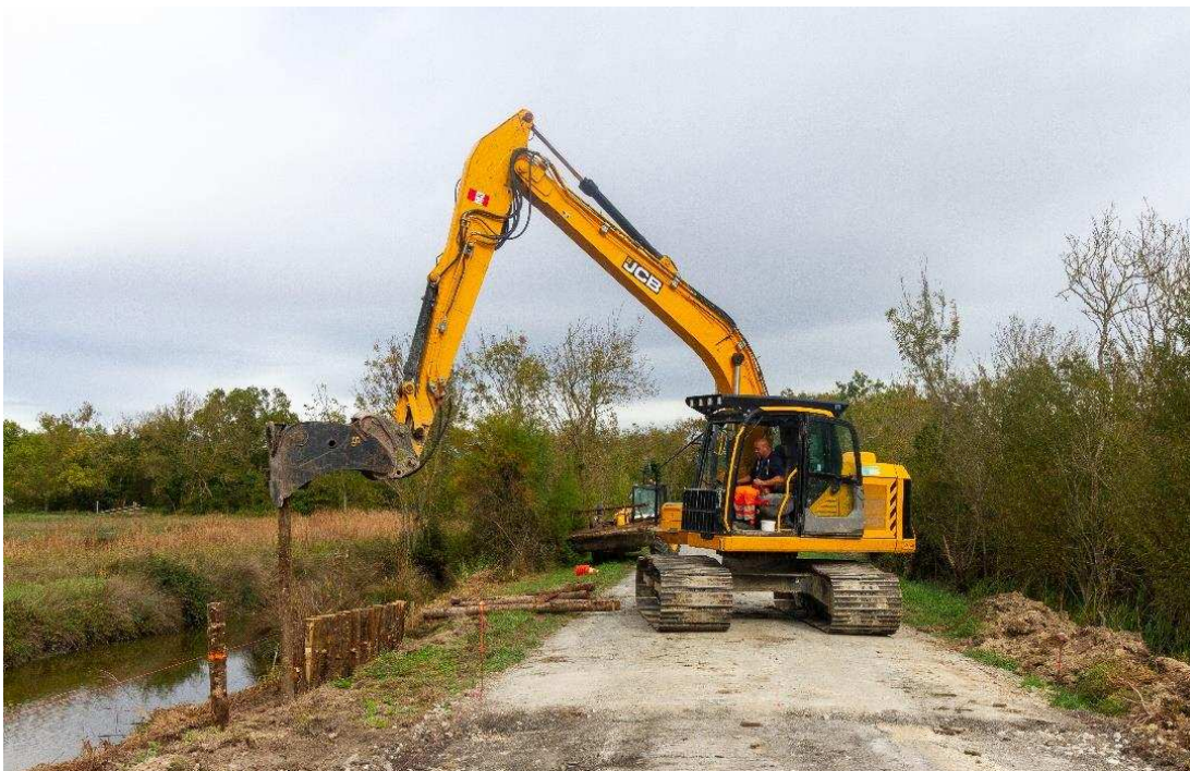
Figure 17: pieutage jointif
