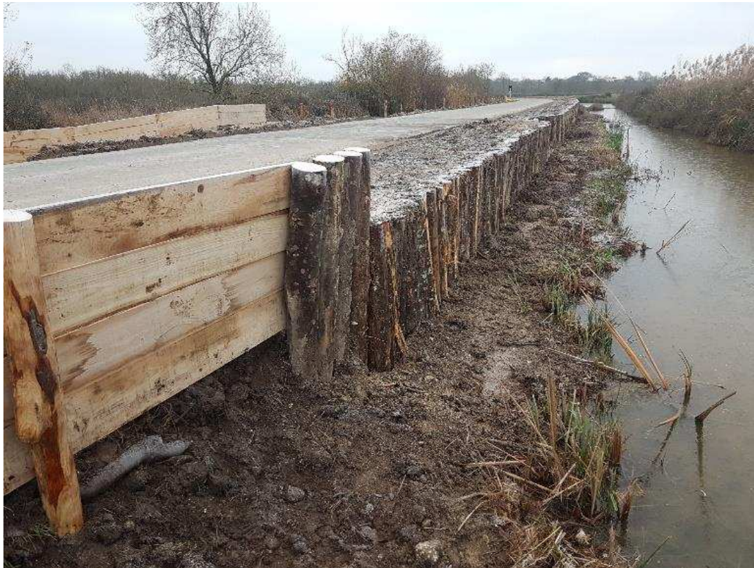
Figure 23: finitions et raccordement au pieutage
