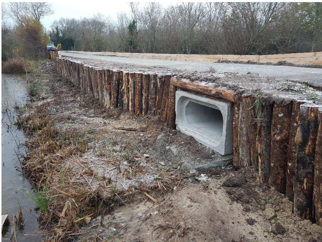
Figure 19: finitions et adaptation aux dalots
