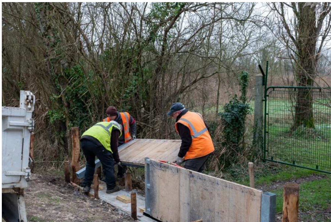
Figure 26: installation des vantaux
